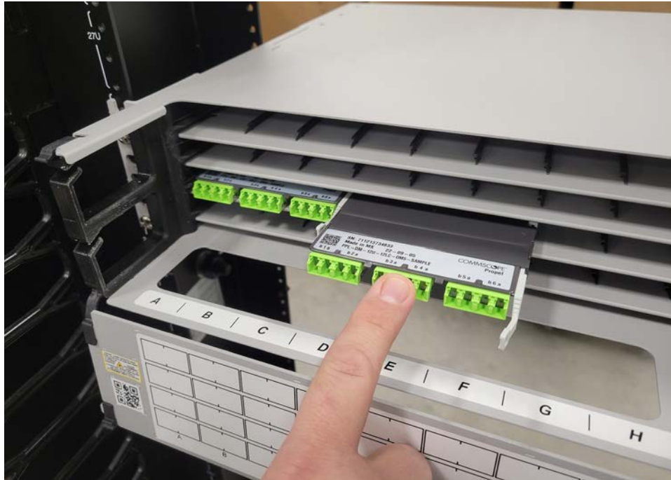
Figure 30. Installing a Connection Component
