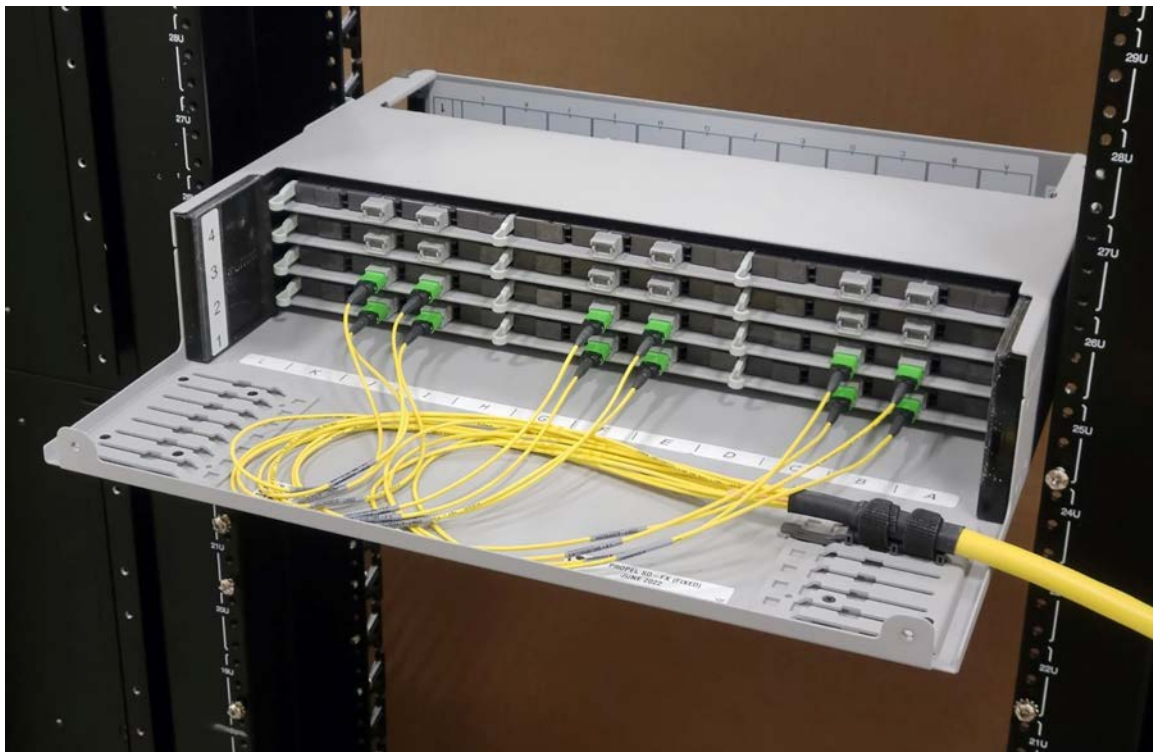
Figure 35. Fully-Installed Cable Assembly with Slack Loop, Propel Fixed Panel
