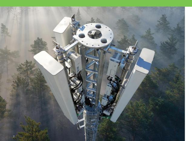
Our next-gen glass fiber reinforced polypropylene (GFRPP) antenna radome is made of 100% recyclable thermoplastic instead of heavier resin and fiberglass designs.
