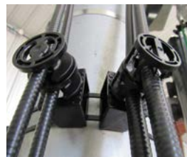
Hangers Installed with SA-1C
