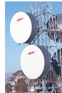
9.16: A typical vertical space diversity arrangement
