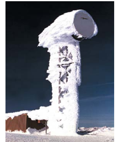
9.14: Ice accumulation on a radome-protected installation
