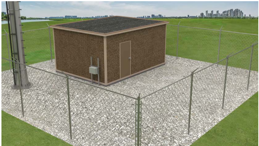
2.6: A traditional cell site enclosure housing radio and base station components
